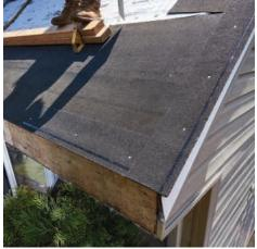
Installs at the eaves and rakes to help prevent shingle blow-off
